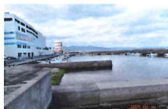
"Youme Town" is being built on the site of the former Kusunoki Port.
